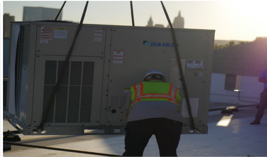
Daikin unit on crane
