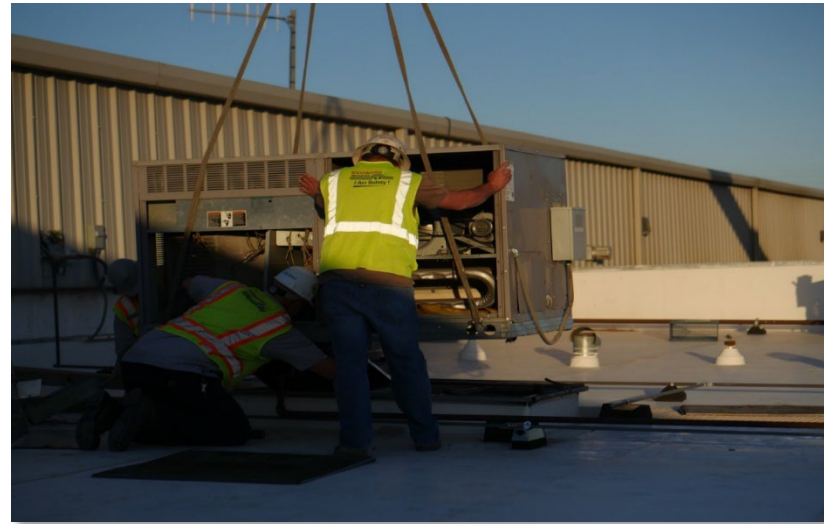
Original unit being lifted off
